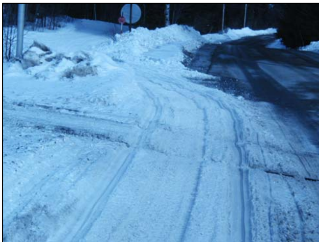
Photo 4.9 Use care to not create snow/ice buildup on railroad tracks
