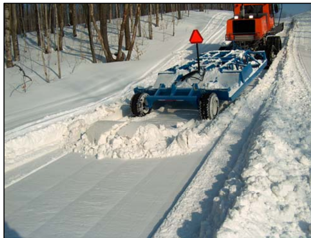
Photo 4.3 Remove back up piles! Use SMV sign.
